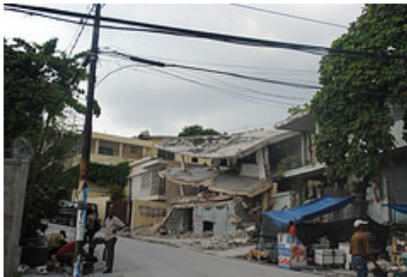
Many streets have been cleared, but over 95% of the rubble remains.
