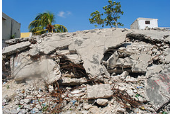
Massive heaps of rubble remain everywhere in the hardest hit areas.
